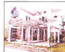
Subdivision Lots with Club- House and Two(2) Unfinished 2 Storey House LA = 14,305.0 sq. m St. Paul Country Homes, Brgy. Sindalan, San Fernando, Pampanga
