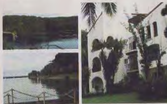
Unit-III Waterfront Condominium Caylabne Bay Resort, Ternate, Cavite FA. 131 P 5,232,000.00
